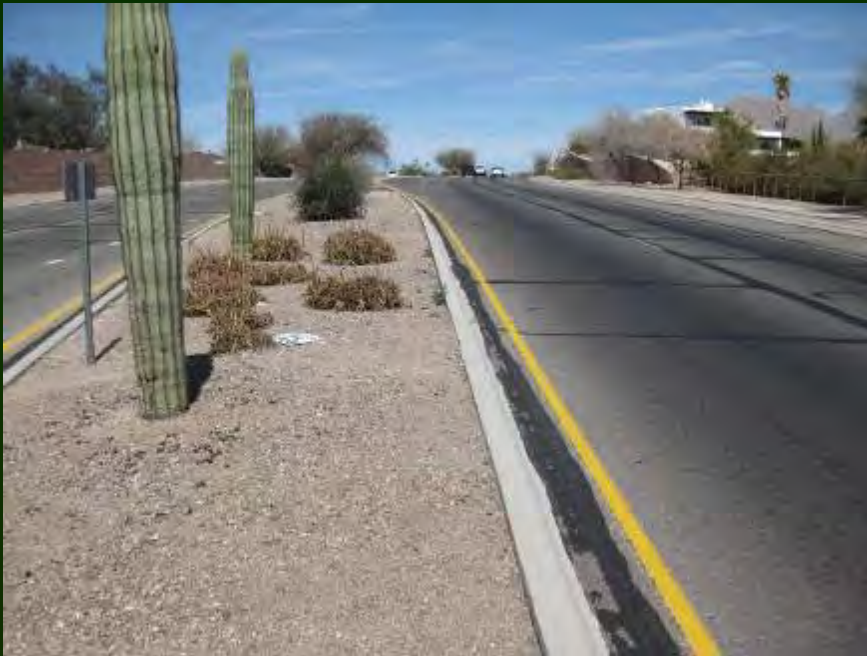
Old design: water collects, causing pavement failure
