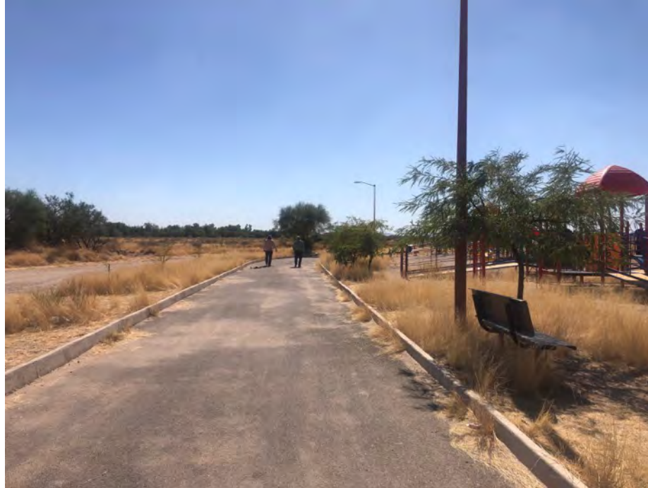
Isolated bikeway lacking maintenance
