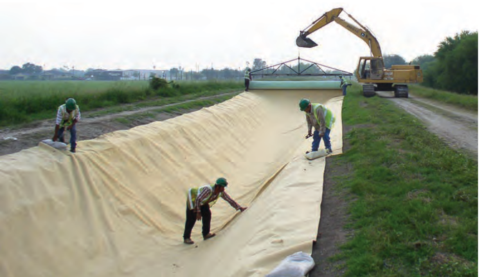
The Lateral “A” Water Conservation Improvements Project in Hidalgo County Irrigation District No. 2 in Texas consisted of placing an impermeable liner along seven miles of concrete canal and protecting the liner with 3 inches of shotcrete. (Certified: June 2003 / Completed: December 2004)
