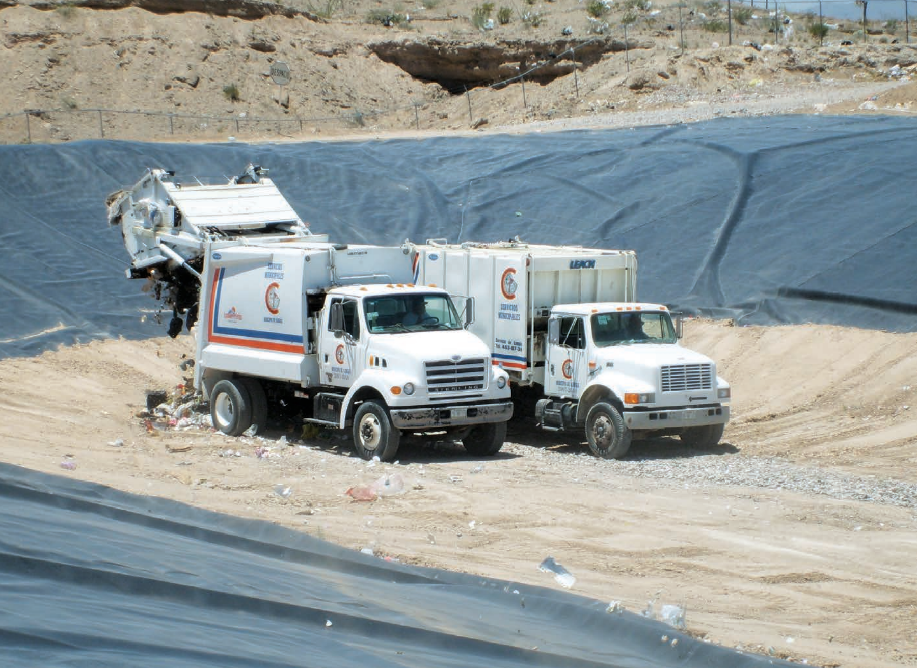
BECC and NADB have supported the construction or expansion of 16 sanitary landfills on both sides of the border, such as this one in Ojinaga, Chihuahua. (Certified: October 2001 / Completed: November 2008)
