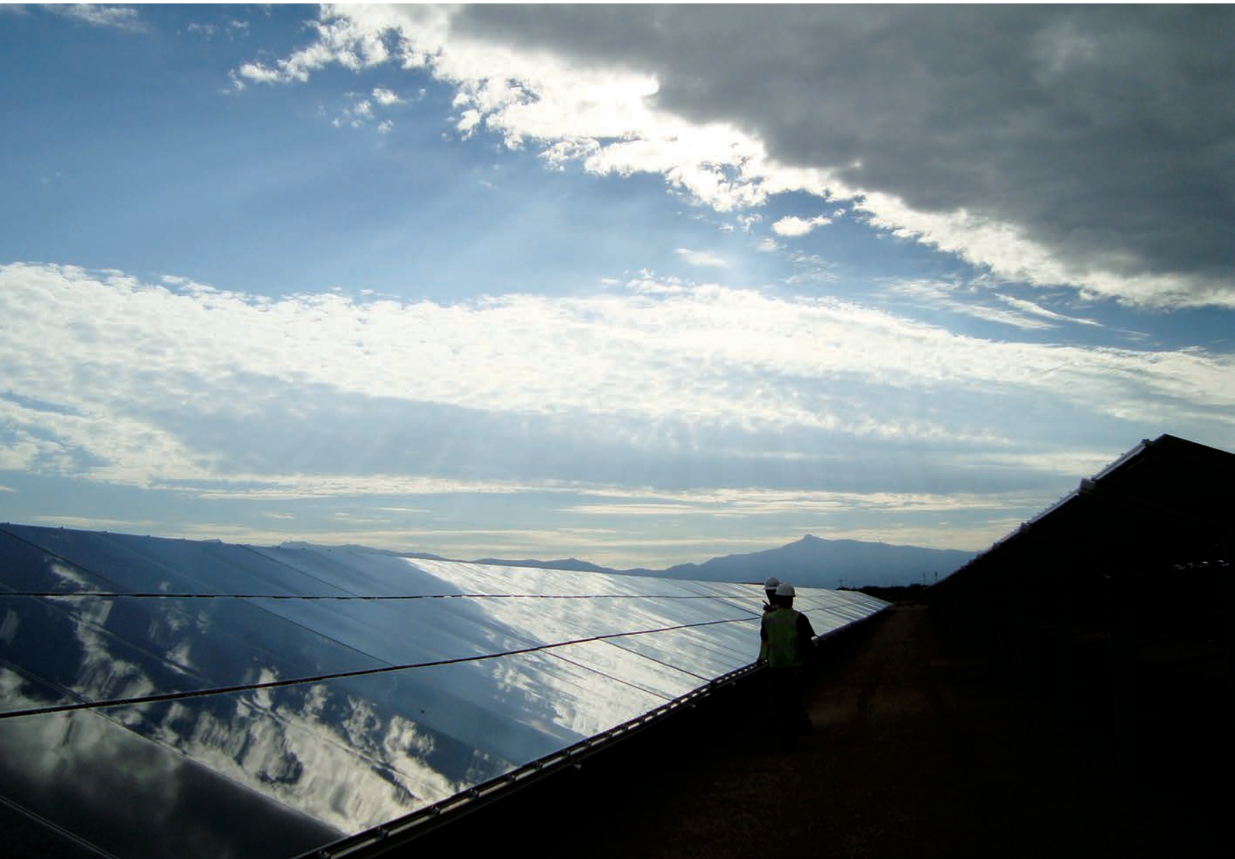
AstroSol Tech Park AZ Project, a 5.1-megawatt solar plant in the University of Arizona Science and Technology Park (UASTP) in Tucson, Arizona. (Certified: January 2012 / Completed: December 2012)
