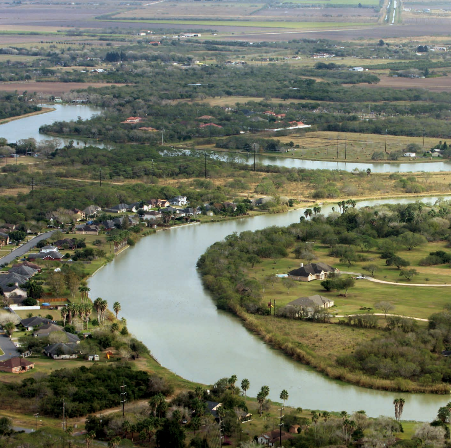
BECC and NADB have supported water and wastewater projects for 13 communities in the Rio Grande Valley of Texas, including the construction or expansion of four wastewater treatment plants with a combined capacity of 7.4 million gallons a day.
