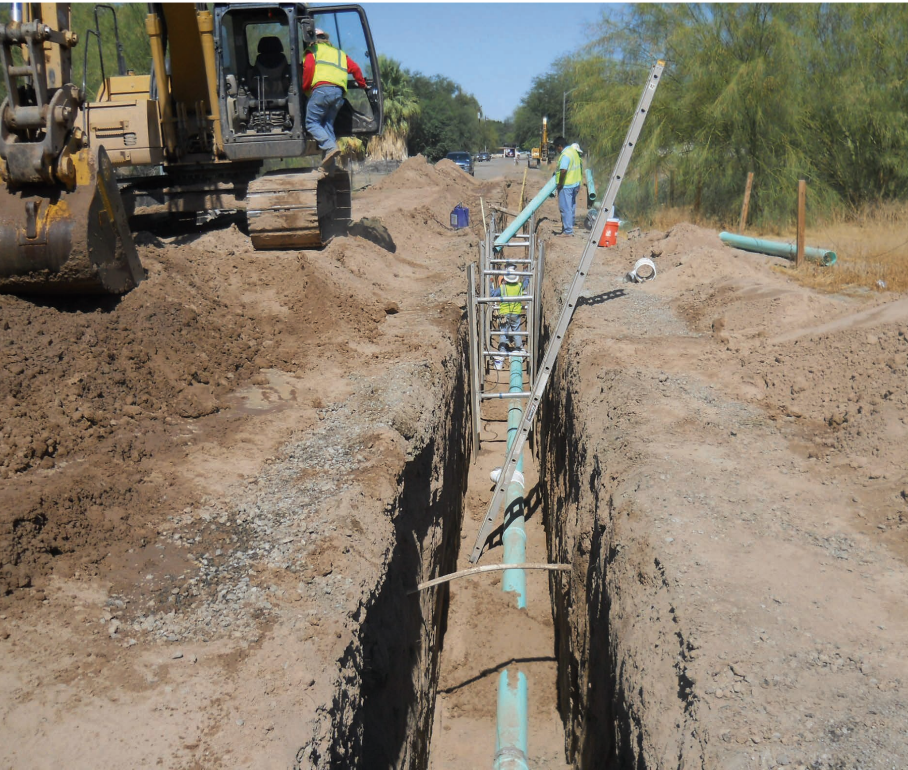
Construction of the Wastewater Collection System for the B & C Colonia in Yuma County, Arizona. (Certified: December 2009 / Completed: February 2012)
