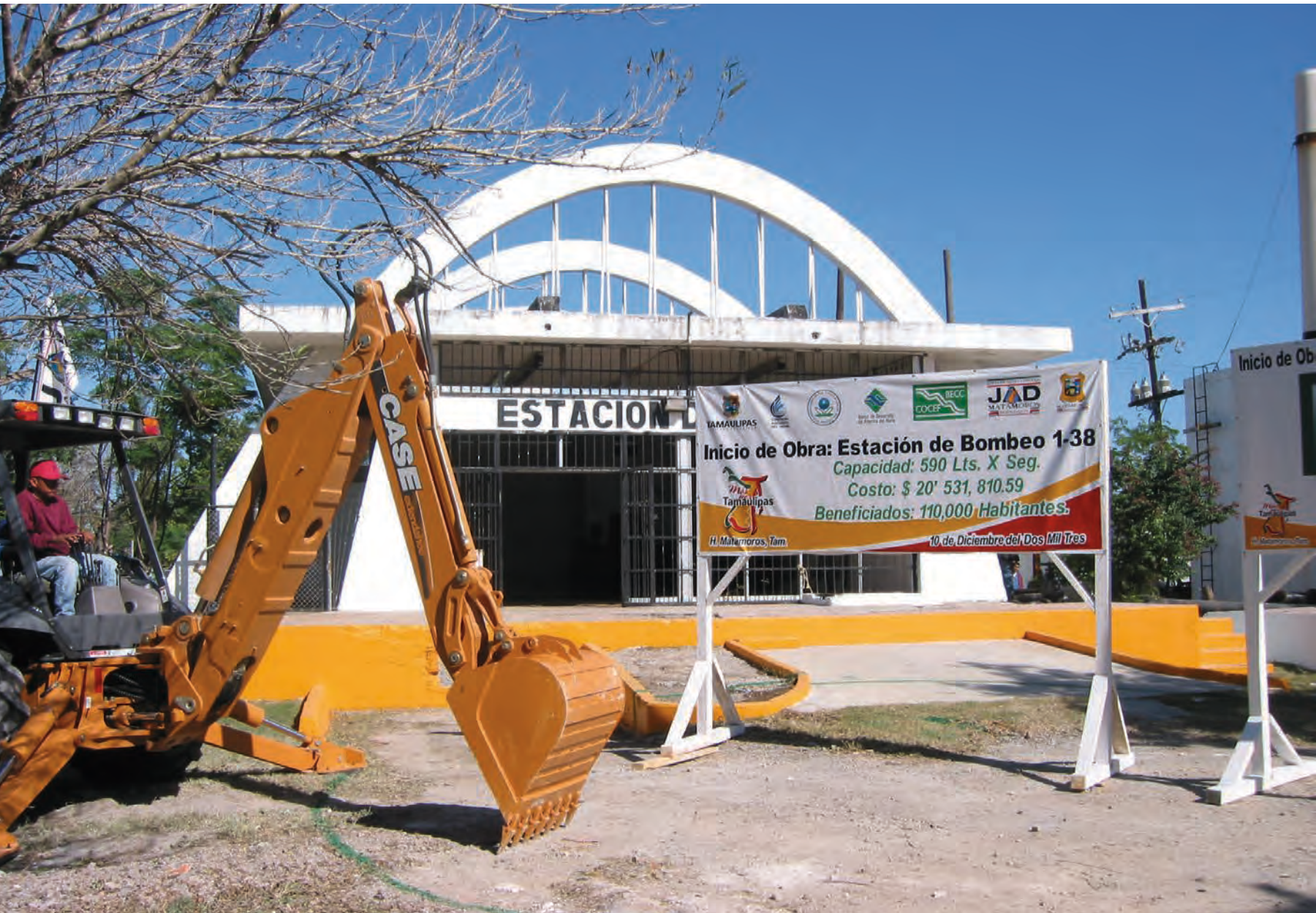
In December 2003 construction began on a new pump station to replace the old infrastructure depicted in the background, as part of the first phase of a comprehensive water and wastewater project in Matamoros, Tamaulipas. (Certified: June 2003 / Completed: September 2008)
