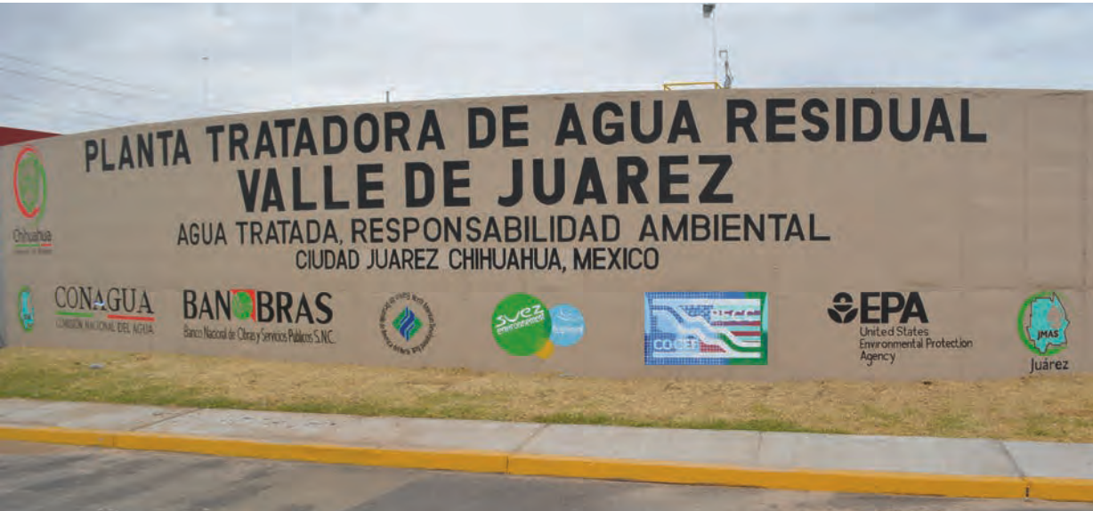
Construction of the South-South Wastewater Treatment Plant in Ciudad Juarez, Chihuahua, is the latest of the four wastewater treatment plants for this border city. (Certified: December 2009)
