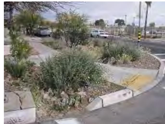
Stormwater management using GI to improve water quality
